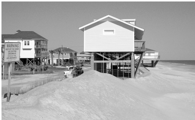
Eroding shorelines threaten beachfront properties, such as this home in North Topsail Beach. Photo: Spencer Rogers
