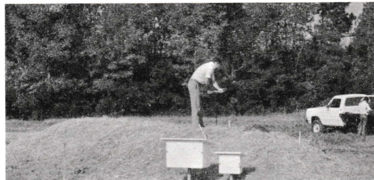
Septic renovation levee: This test system serves two houses in Plymouth, N.C. It is three feet high and 50 feet long.
