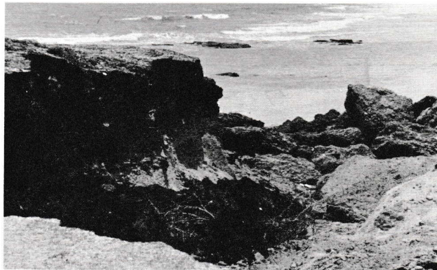
Remains of a former U.S. Highway 421, washed out by erosion.
