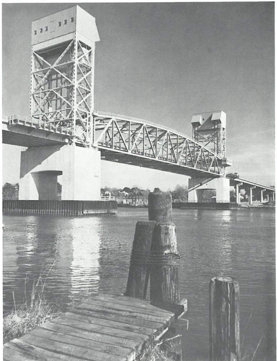
Cape Fear Memorial Bridge near Wilmington
