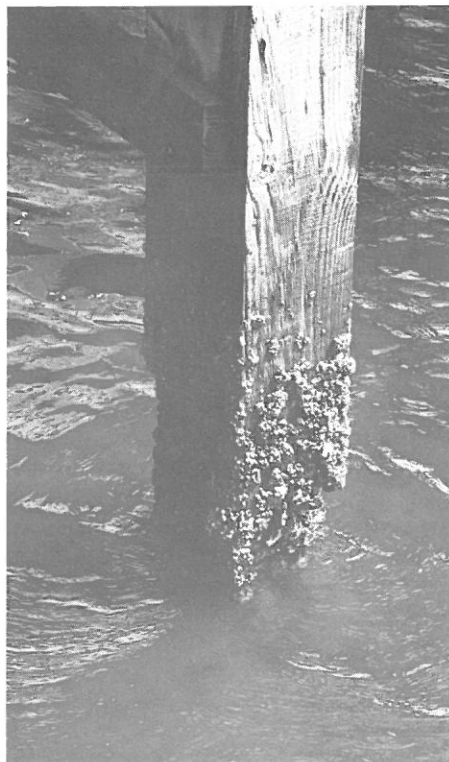
Dry-stack marinas like this one near Atlantic beach store many boats efficiently. But at any saltwater marina, maintenance is a problem. Damaged pilings like the one at right, from a marina near Morehead City, must be replaced before the structure becomes unsafe.
