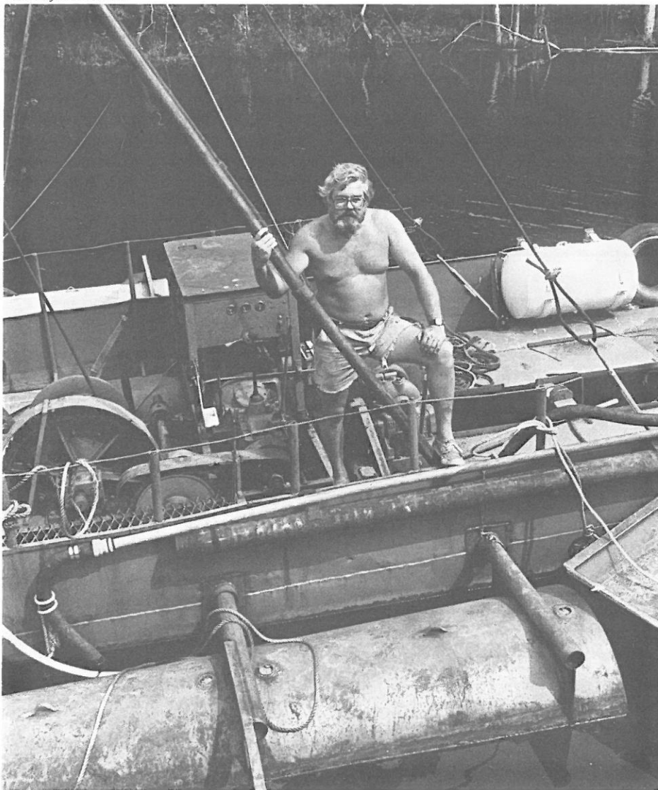
Keith Wolfenbarger on his pile driver
