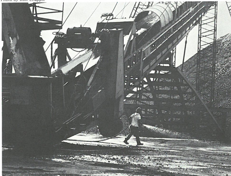
Workmen use water hoses to control dust at the terminal
