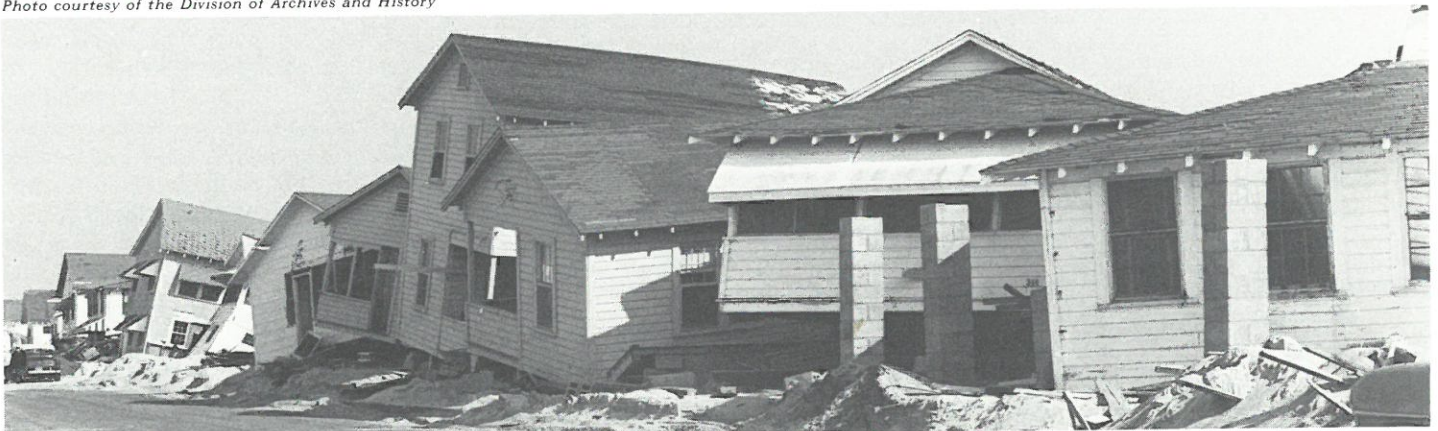
A row of houses lie toppled like building blocks at Carolina Beach one month after Hazel
