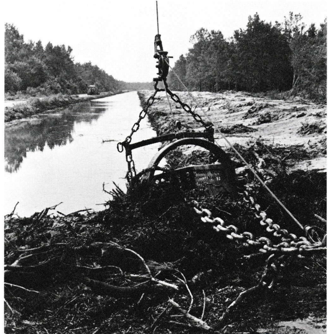
Drainage canal under construction
