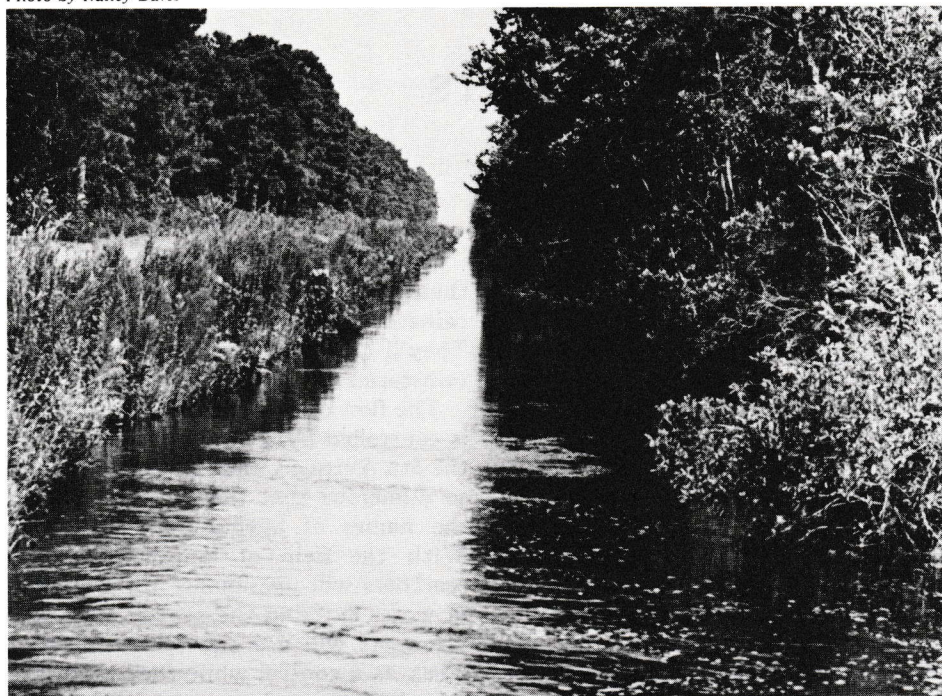
5th Avenue Canal carries water from ditches to the sound
