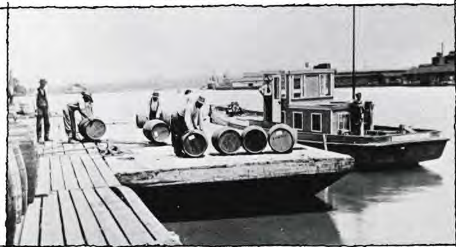
Workers load naval stores on a wharf at Eagles Island.
