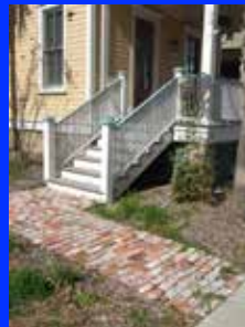
Old Brick Pavers for Sidewalks
