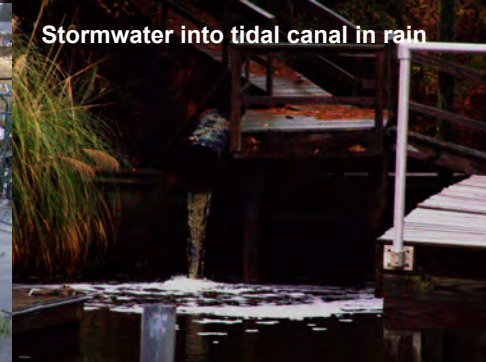
Suburban storm drain directly into canal, canals receive fecal bacteria, nutrients, metals, PAHs from auto / boat fuels and oil into a poorly flushed area
