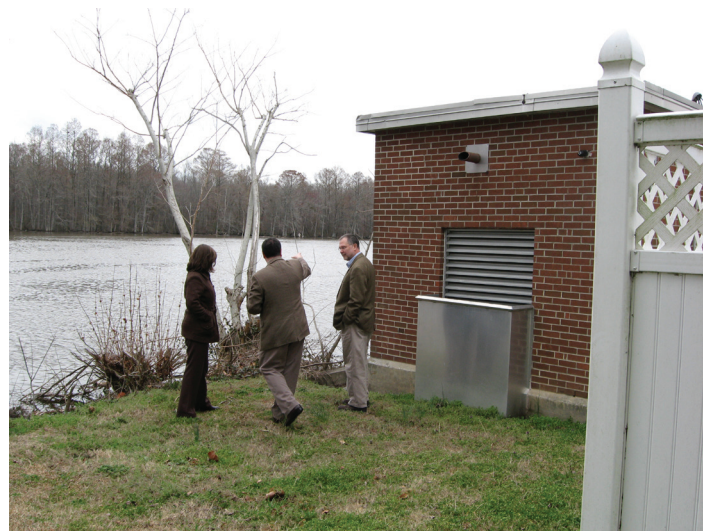
Pumping station adjacent to Roanoke River
