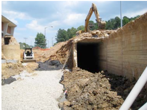
Prior to Phase III, Rocky Branch flowed through this concrete culvert. It took construction crews
