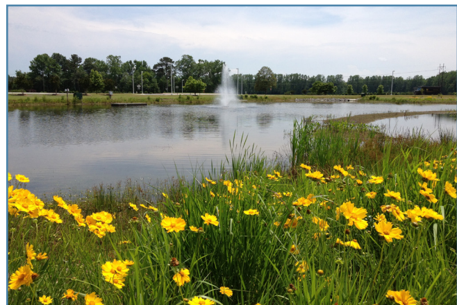
Wetland benches, floating treatment wetlands and perimeter plantings can be added to stormwater ponds to improve both treatment and aesthetics. (Natalie Carmen, Dept. of Biological and Agricultural Engineering, North Carolina State University)
