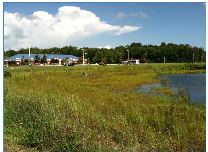
After two growing seasons, vegetation is becoming established on a wetland bench added to the stormwater pond in front of the Currituck County Cooperative Extension building. (Photo: North Carolina Sea Grant)
