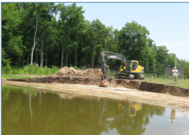
The wetland bench is added to the perimeter of an existing pond by removing soil using an excavator. (Photo: North Carolina Sea Grant)
