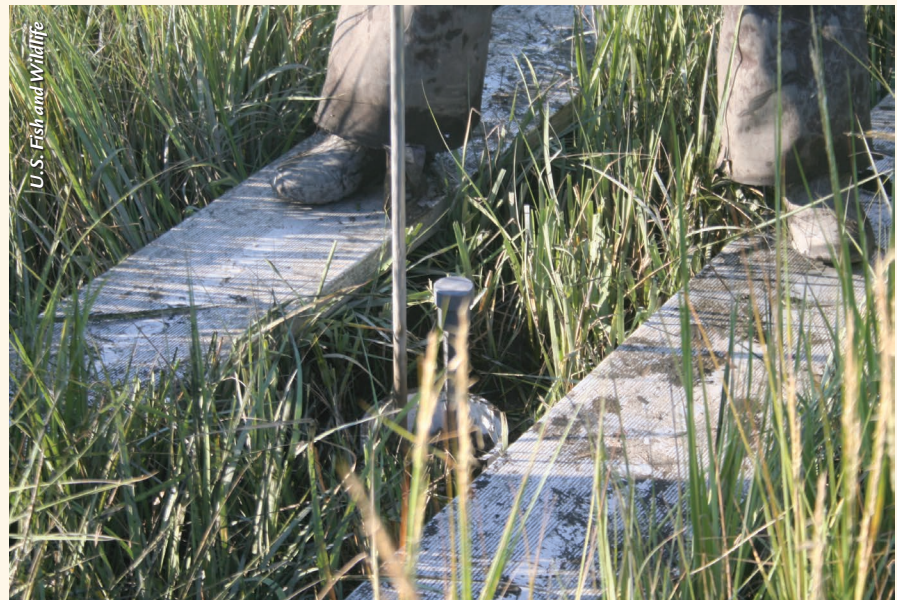
SET ROD INSTALLATION.
