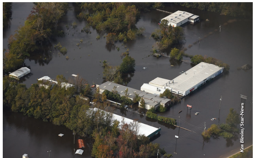
Flooding from the Neuse River near Kinston.
