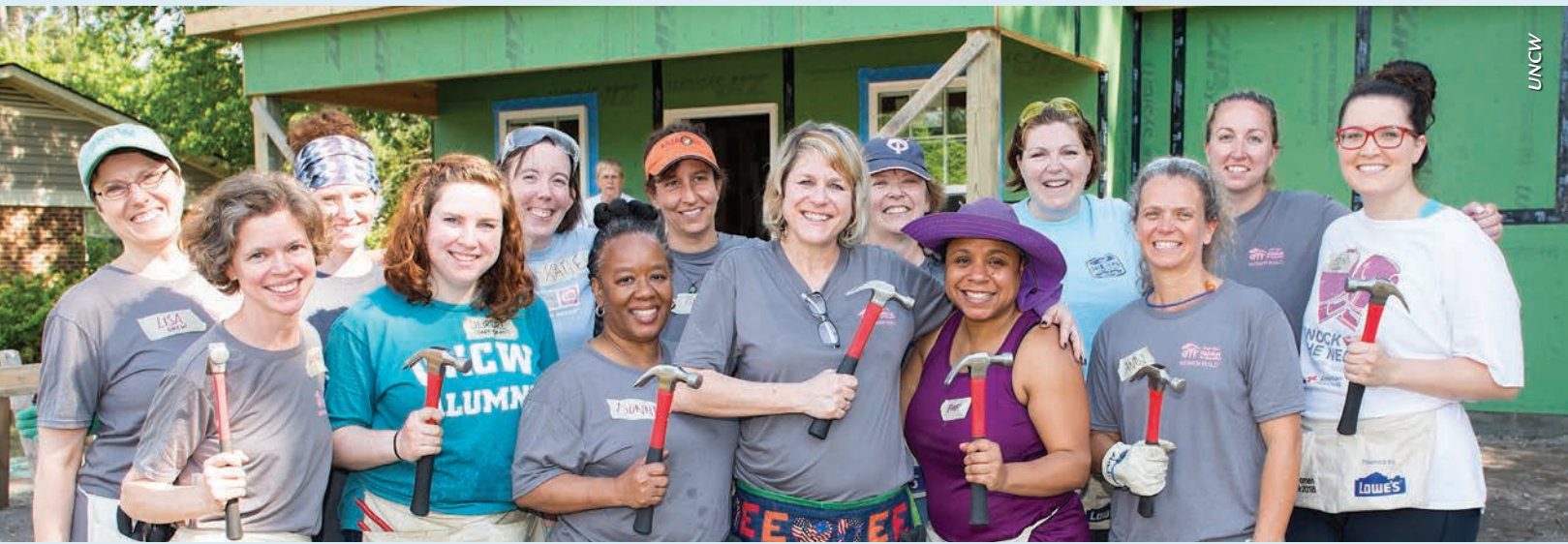
Habitat partnered on a FORTIFIED home construction with Katherine Montwieler (front row, far left) and UNCW's Women Build team (shown here on an earlier project).
