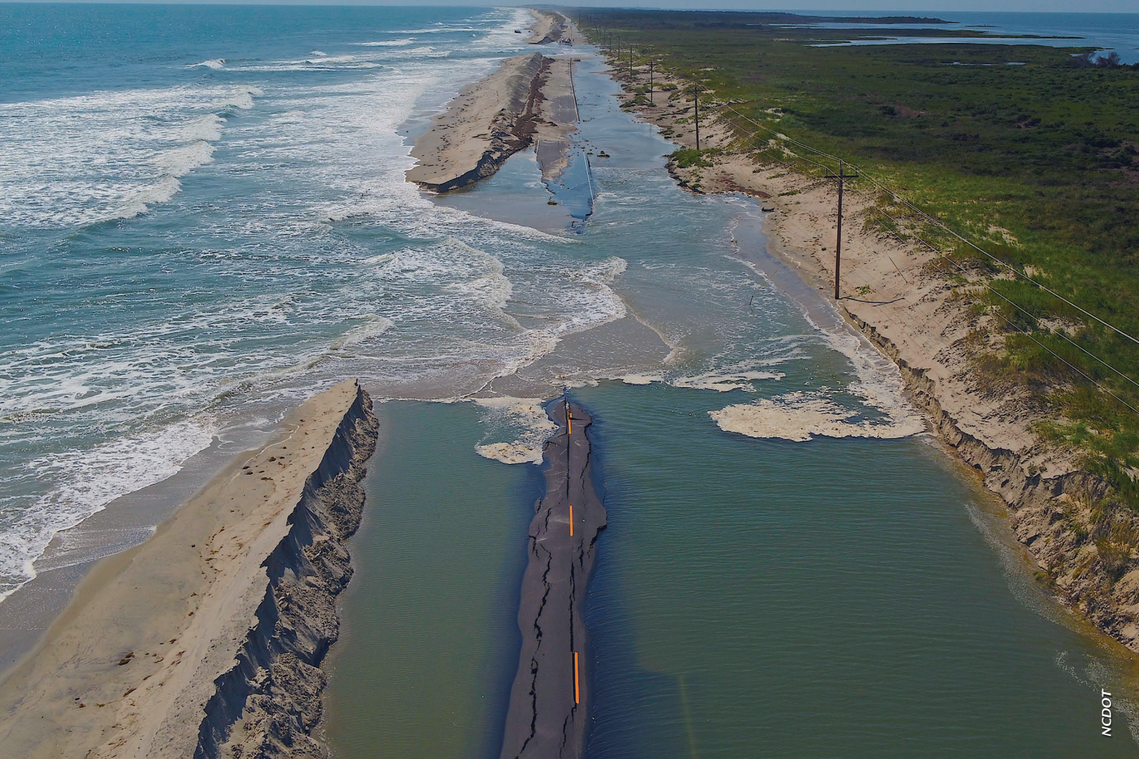
Catastrophic flooding across NC Highway 12 on Ocracoke Island after Hurricane Dorian in 2019.
