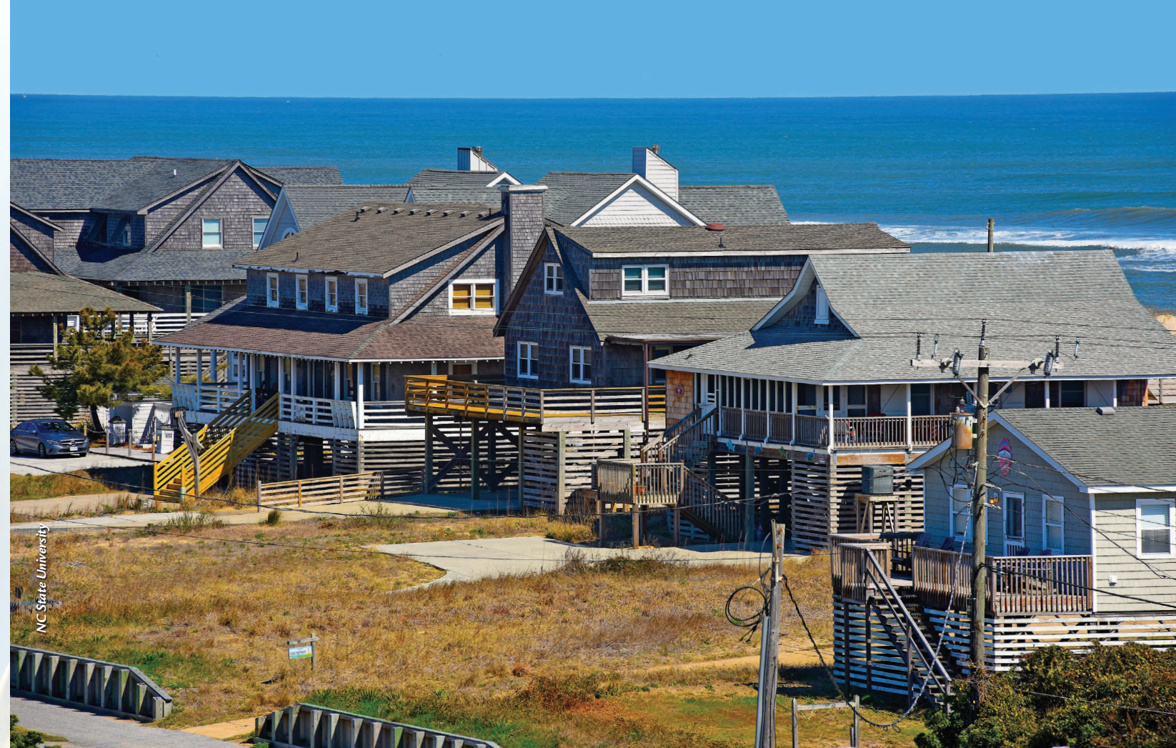
NAGS HEAD IS MOVING AHEAD WITH A PIONEERING WASTEWATER MANAGEMENT PLAN, WHICH INCLUDES A SUITE OF RECOMMENDATIONS THAT INCORPORATE RESEARCH FROM JANE HARRISON'S SEA GRANT TEAM, AS WELL AS FROM OTHER SOURCES.
