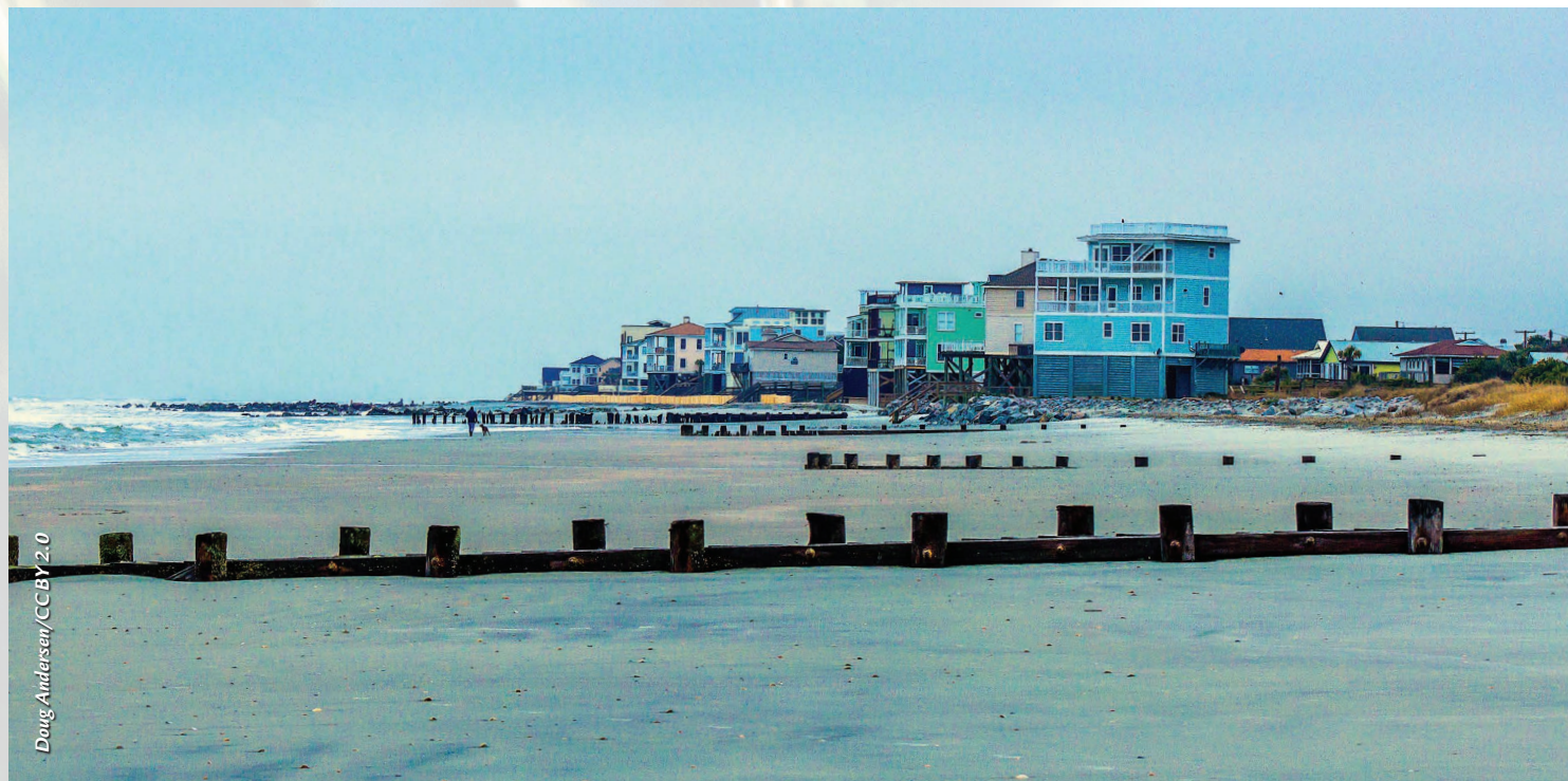
THE COMMUNITIES OF NAGS HEAD (ABOVE) AND FOLLY BEACH (BELOW) ARE PARTNERING ON A SEA GRANT PROJECT THAT ADDRESSES THE CHALLENGES THAT RISING SEAS POSE FOR WASTEWATER TREATMENT.
