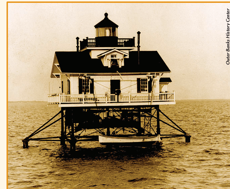
• ABOVE: THE ROANOKE MARSHES SCREW-PILE LIGHTHOUSE STOOD AT THE SOUTH ENTRANCE TO CROATAN SOUND ON AN ERODING MARSH ISLAND FROM 1867 TO 1955.
