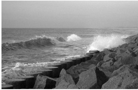
The construction of a seawall in 1996 to protect Fort Fisher, a State historic site, increased erosion at a nearby development called The Riggings. Photo: Spencer Rogers
