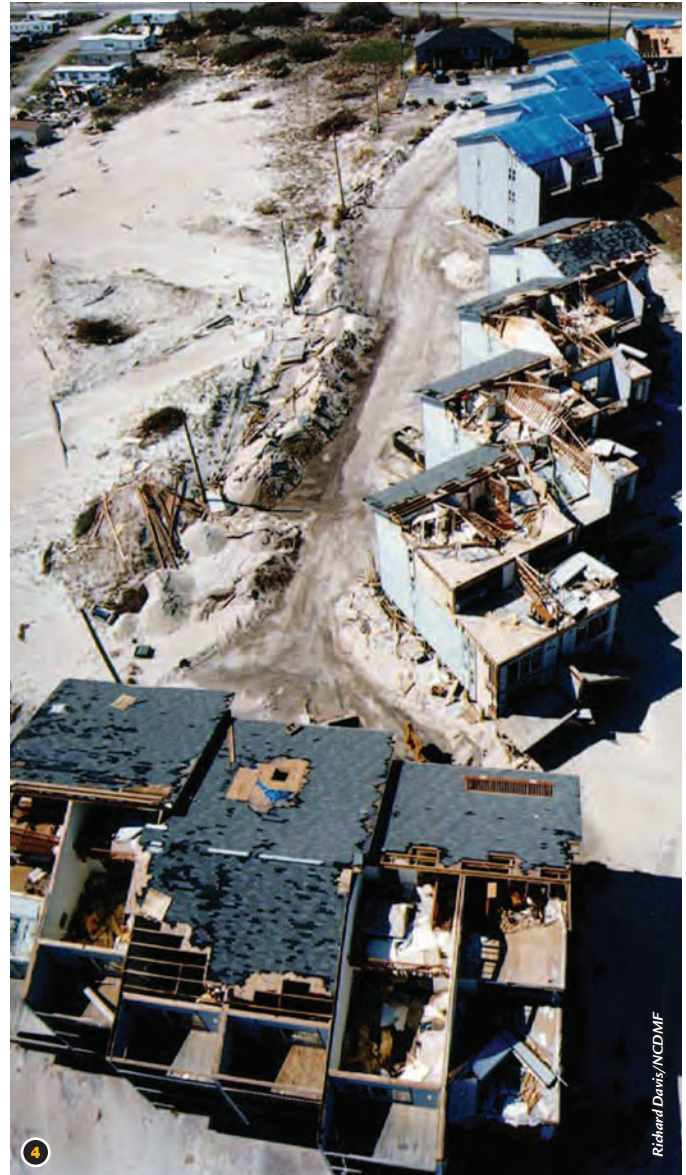
1. Elevating a home is one way to protect the structure from storm surge, waves and flooding. 2. Homes on North Topsail Beach that adhered to building codes implemented after 1986 weathered Fran fairly well. 3. Storm surge and waves from Fran exposed pilings in coastal homes. 4. Fran brought water, sand and wind damage to these homes in Surf City.
