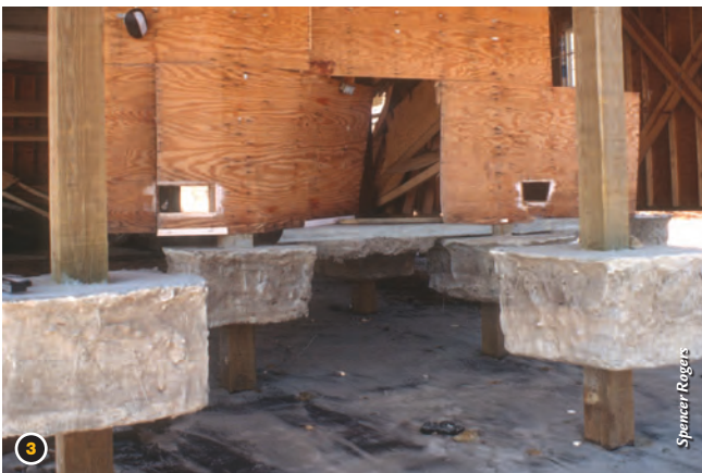
1. Elevating a home is one way to protect the structure from storm surge, waves and flooding. 2. Homes on North Topsail Beach that adhered to building codes implemented after 1986 weathered Fran fairly well. 3. Storm surge and waves from Fran exposed pilings in coastal homes. 4. Fran brought water, sand and wind damage to these homes in Surf City.
