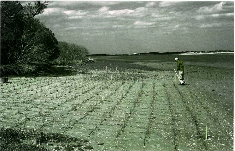
Figure 1. Transplanted salt marsh grasses are an alternative erosion-control method.
