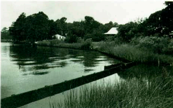
Figure 7. An offshore breakwater, in combination with a planted marsh, can provide long-lasting erosion protection at relatively low cost.
