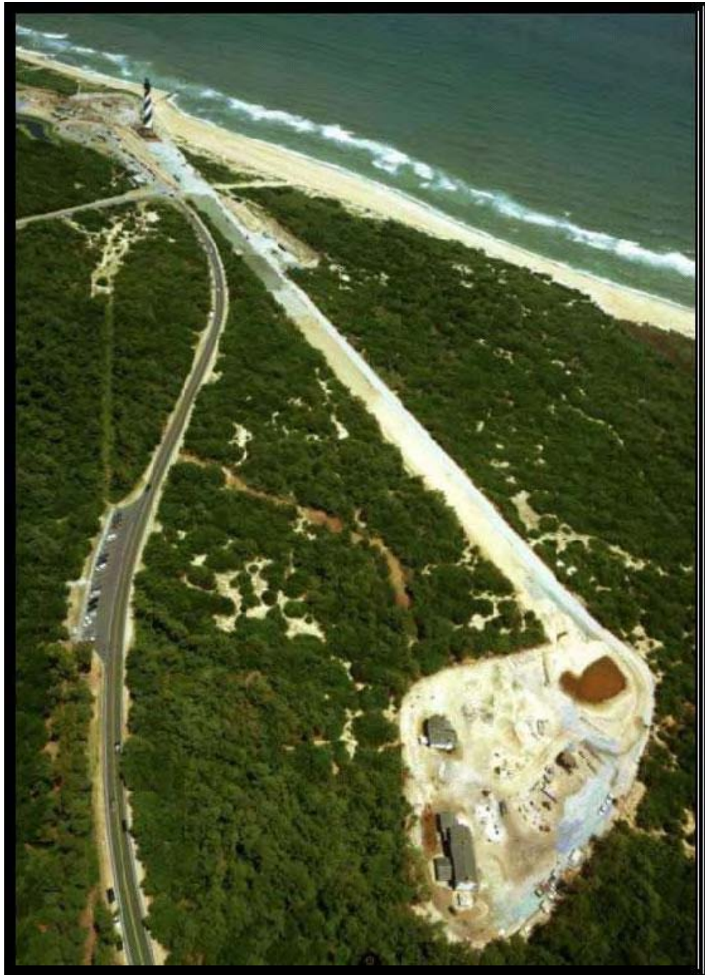
Figure 1-33. Cape Hatteras Lighthouse is being prepared for its move from the old threatened site adjacent to the rapidly eroding shoreline to a new inland site. Photograph is by the N.C. Department of Transportation.
