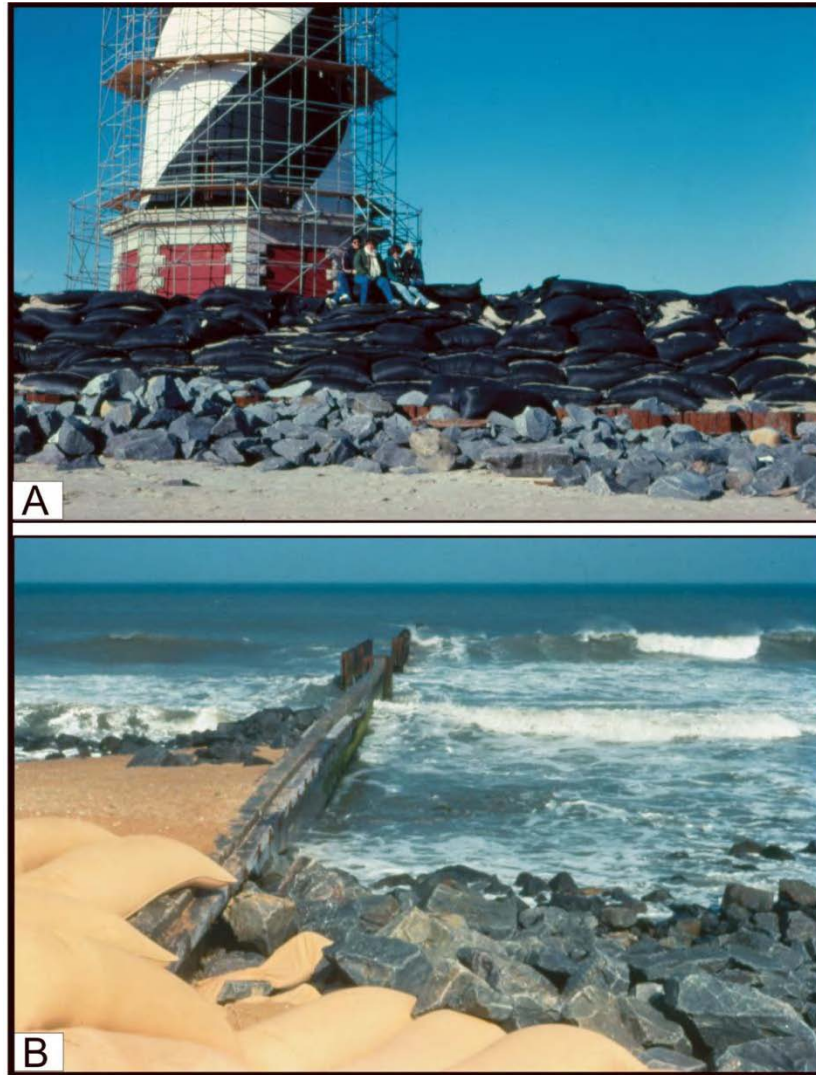
Figure 1-32. Panels A and B. Photographs of the extensive effort to protect the Cape Hatteras Lighthouse from the encroaching Atlantic Ocean with massive hardened structures. These photos show a steel bulkhead, a steel groin, several rock revetments, and many layers of sand bags that have been used over decades in desperate attempts to “hold the line.” Photographs are by S. Riggs.
