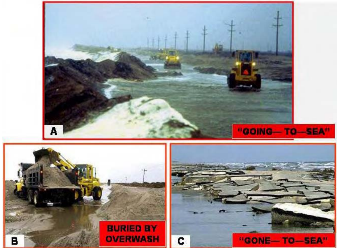
Figure 2-12. N.C. Hwy. 12 “going-to-sea” as the storm tide washes over the road during a typical nor’easter. In some storms the highway is just buried in overwash sand that is cleared off the road and put back into a barrier-dune ridge. Other storms physically destroy the road as it finds itself in the surf zone. Photograph A is by O.H. Pilkey, B is by S. Riggs, and C is by Cape Hatteras National Seashore personnel.
