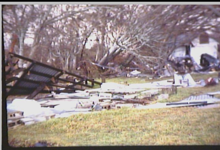
Figure 42: Hurricane damage on the Carolina coast.
