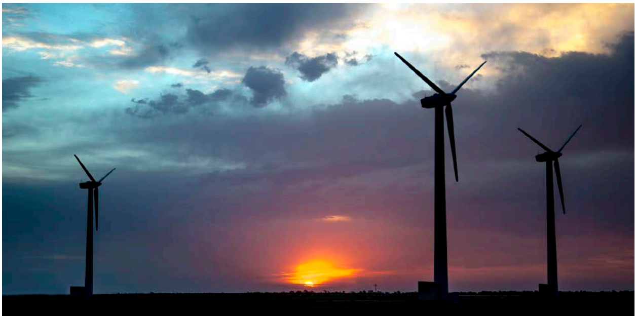
The Department of Energy/Sandia Scaled Windfarm Technology facility in Lubbock, Texas. Photo by Lloyd Wilson/SandiaLabs.
