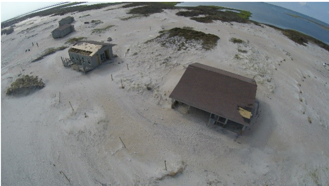
Overwash and damage from Hurricane Florence to cabin facilities at Great Island. Photo courtesy of CALO NS.
