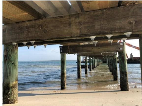
New cross members, beefier stringers and attachment hardware, and hog-slats on the Shackleford Banks pier and dock. Photo courtesy of CALO NS.
