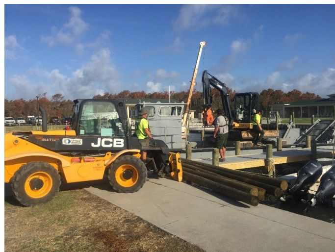
After Hurricane Florence, NPS staff replaced pilings, raised docks and replaced decking with thru-flow composite material. Photo courtesy of CALO NS.
